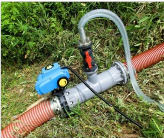
Picture 3 Connection part of inlet pipe of Siphon Intake
