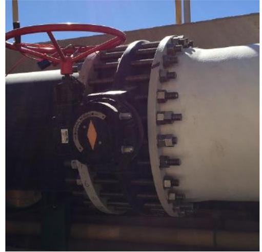
Photo 3 Butterfly Valves have been employed in mines in South America
