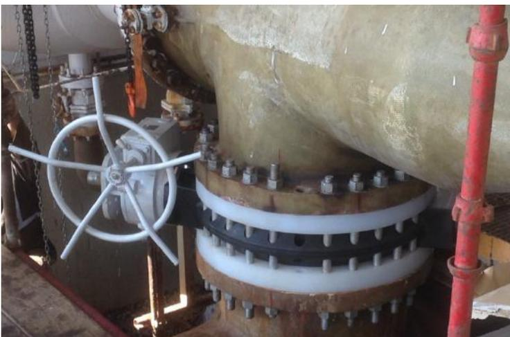
Photo 6 they were replaced with Butterfly Valve Type 58
