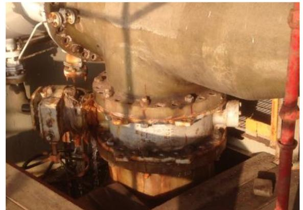
Photo 5 Using metal valves caused external leakage
